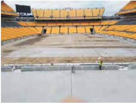
View from top of the new Heinz Field seats
